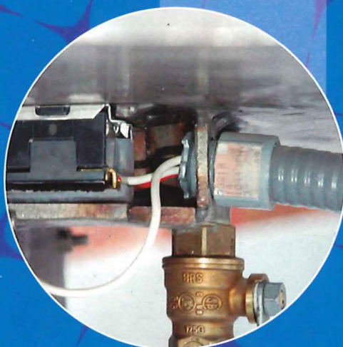
THERMOSTAT & GROUND WIRE.
